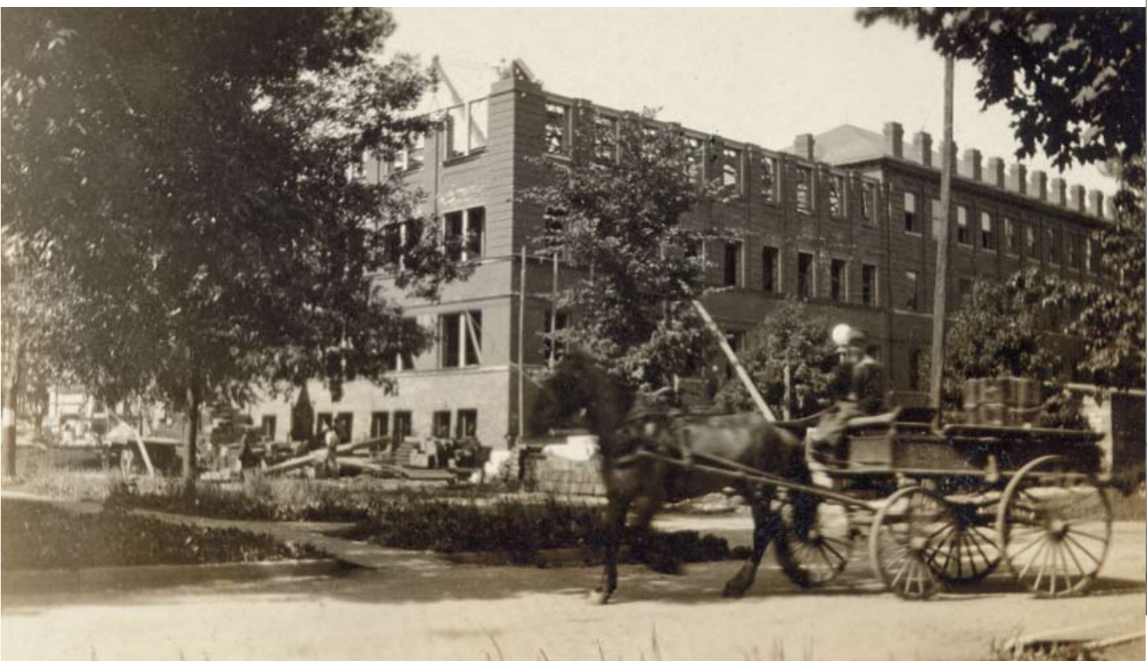
Construction of Noyes Laboratory, circa 1916.
